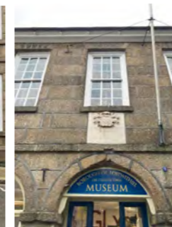
Fore Street Elevation of Museum / Guildhall
