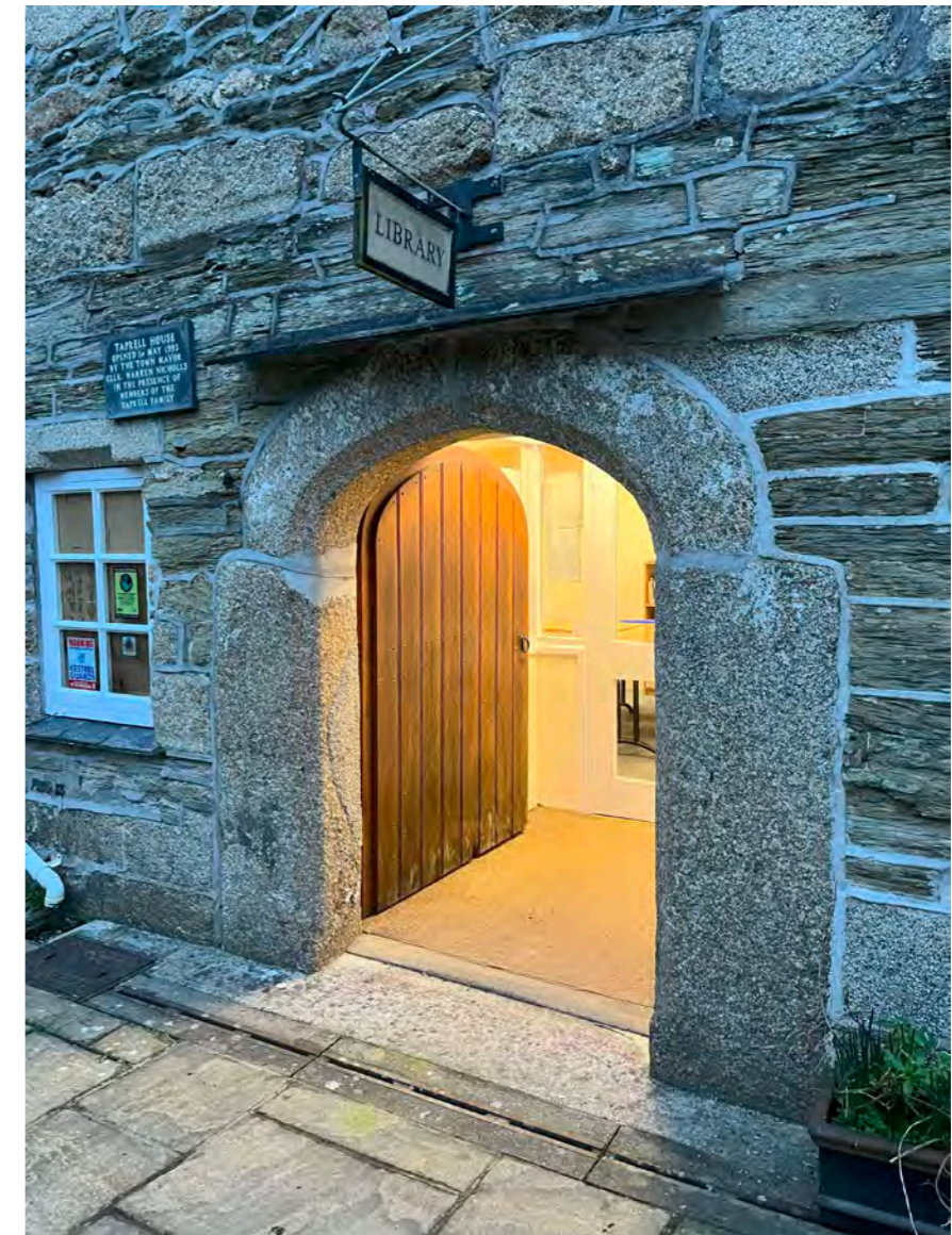
Current entrance into Taprell House
