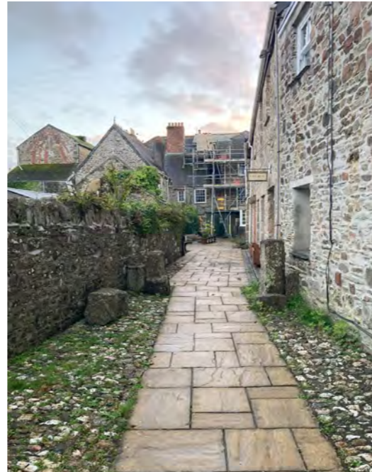
Entrance alley to Taprell House from North Street
