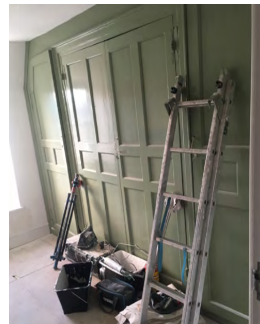
Recently redecorated internal joinery
