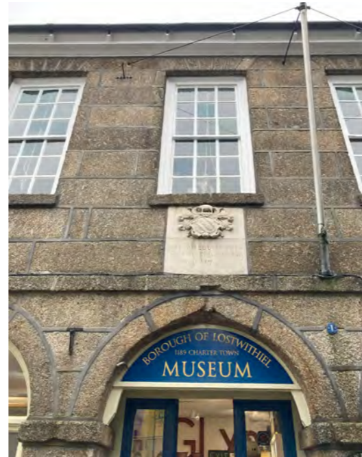
Fore Street elevation of Museum / Guildhall
