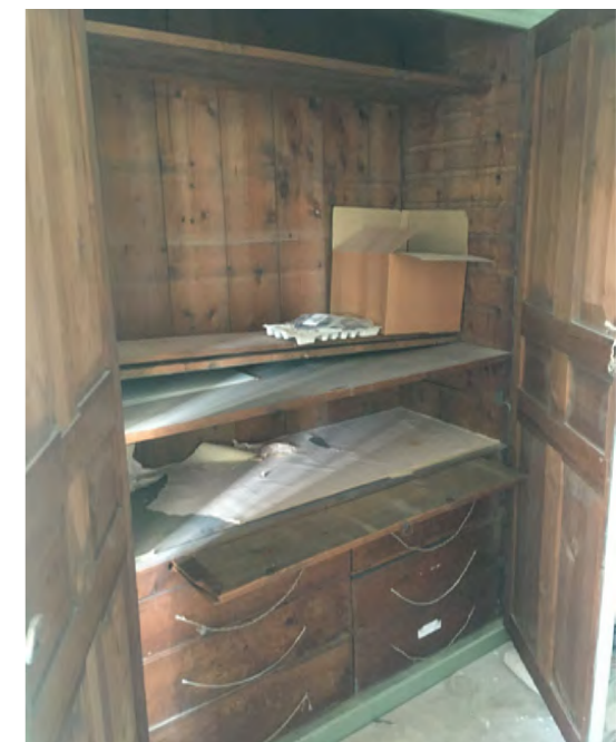
Existing internal joinery
