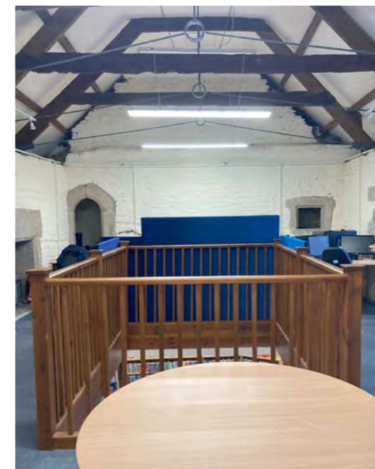
View of mezzanine area in Taprell House
