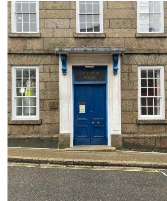
Fore Street entrance to Edgumbe House
